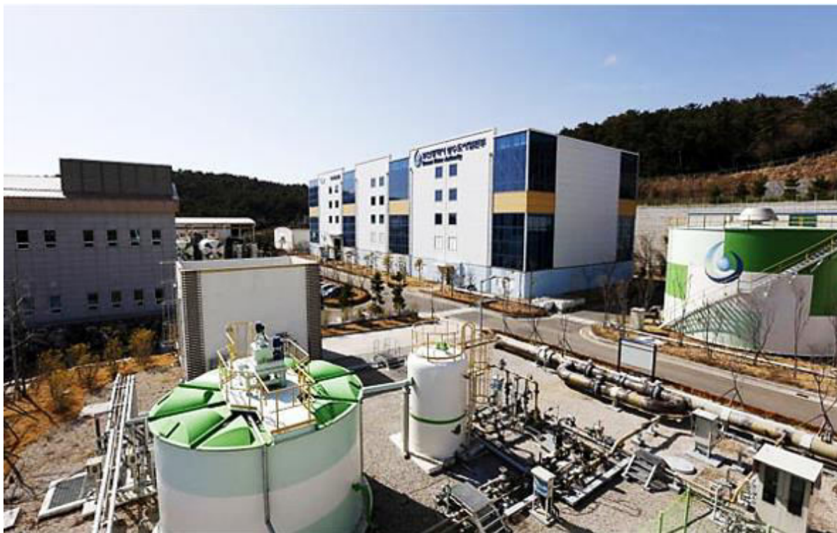
Fig. 1: Gijang seawater desalination facility.
